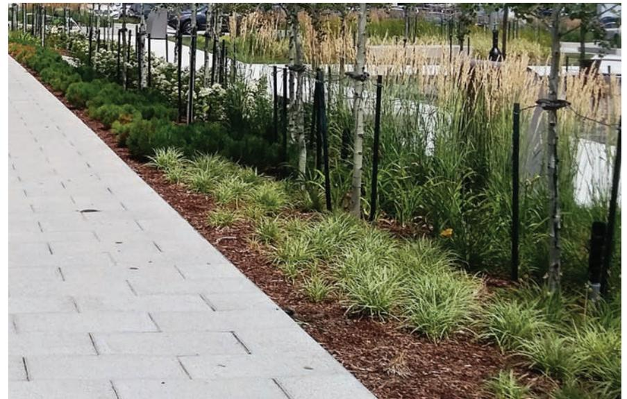
Low impact development that minimizes impact of stormwater run-off.
