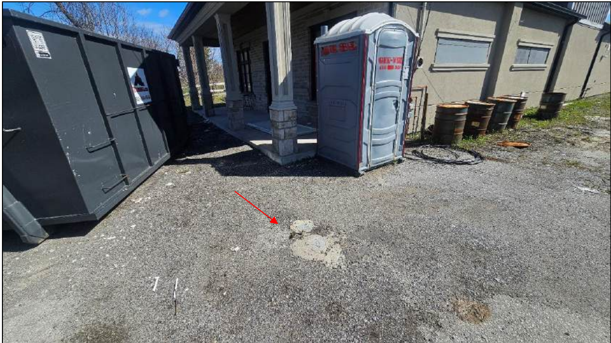
Photograph 9: Representative view of monitoring wells at 12371 Highway 8.
