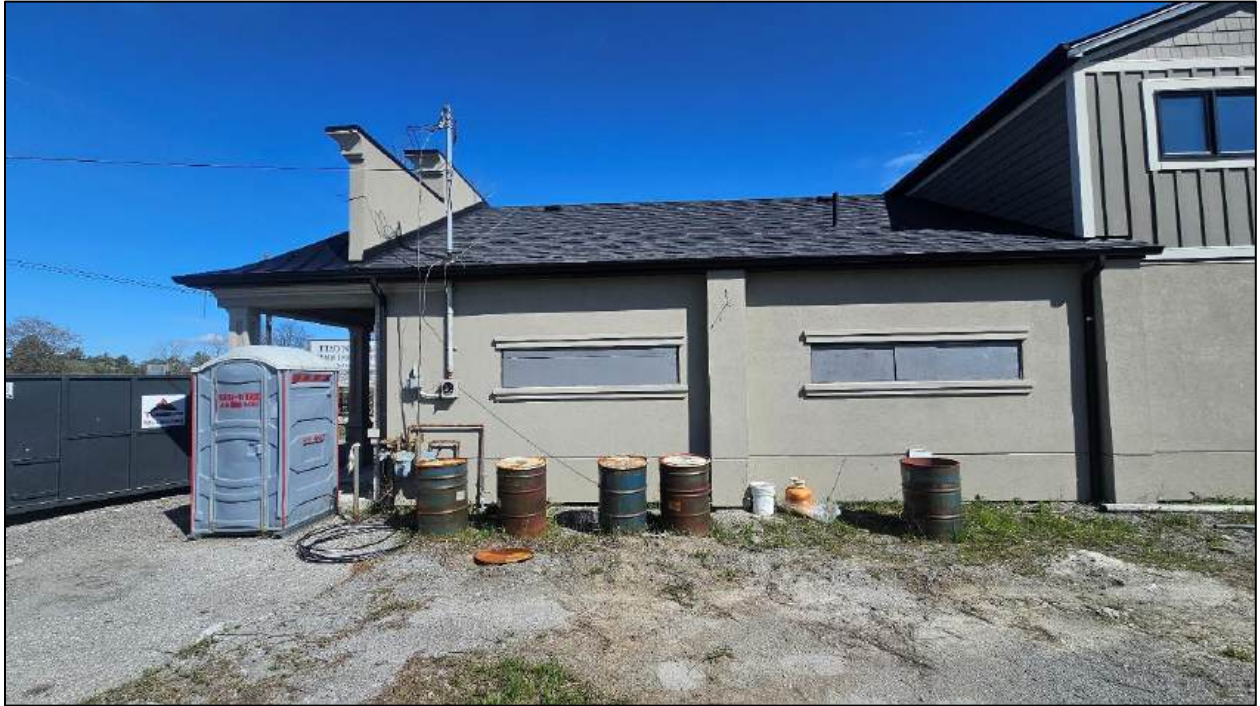
Photograph 15: View of soil cutting drums observed at 12371 Highway 8.
