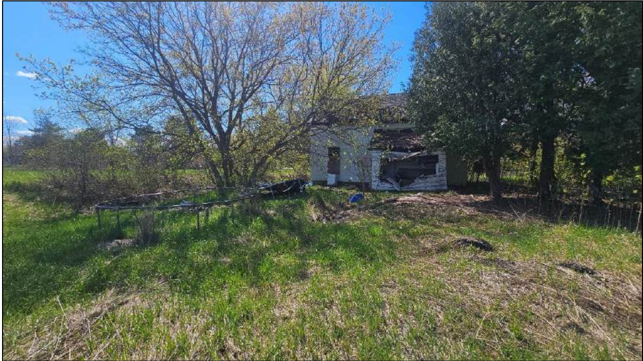
Photograph 5: View of the residential Site building at 5318 Main Street (facing south).
