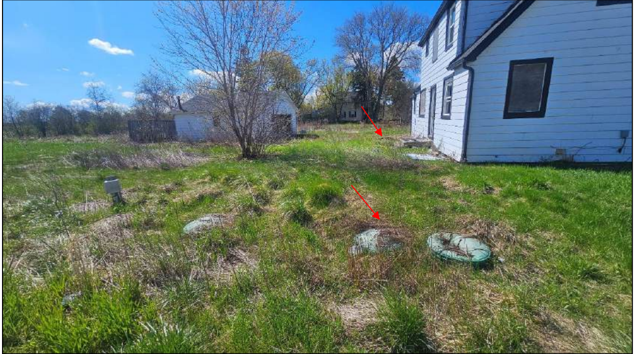
Photograph 13: View of septic pit and bed at 12371 Highway 8.
