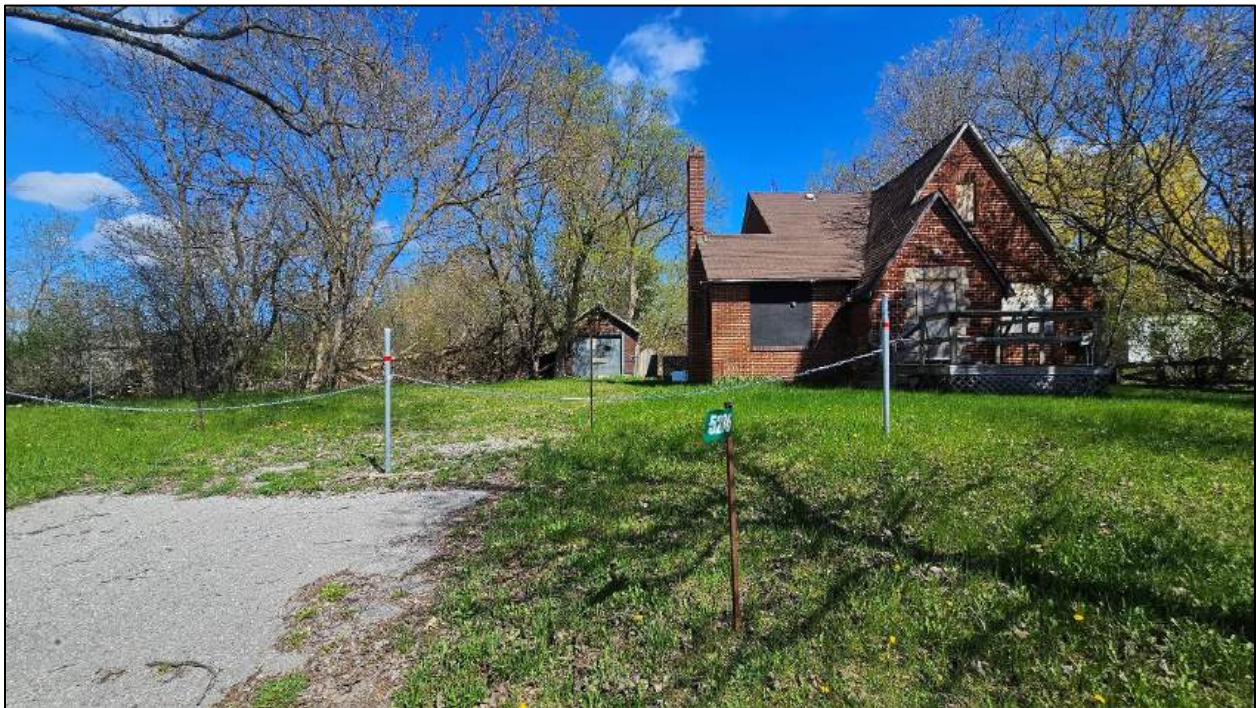
Photograph 4: View of the residential Site building at 5286 Main Street (facing north).
