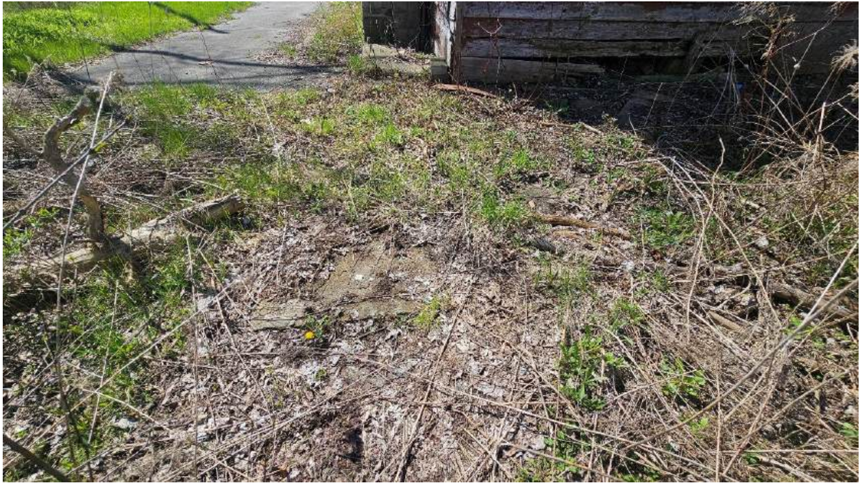
Photograph 17: View of inferred septic pit with concrete slab at 5270 Main Street.
