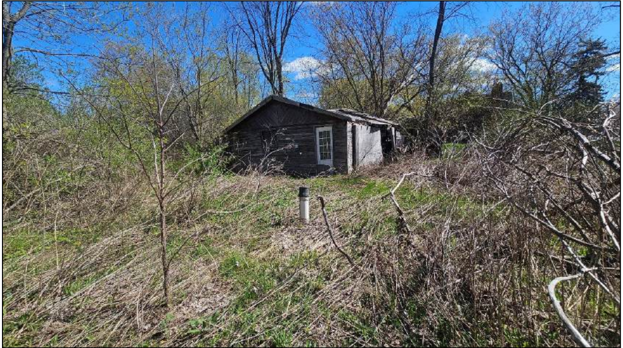
Photograph 11: View of capped water well at 5270 main Street.
