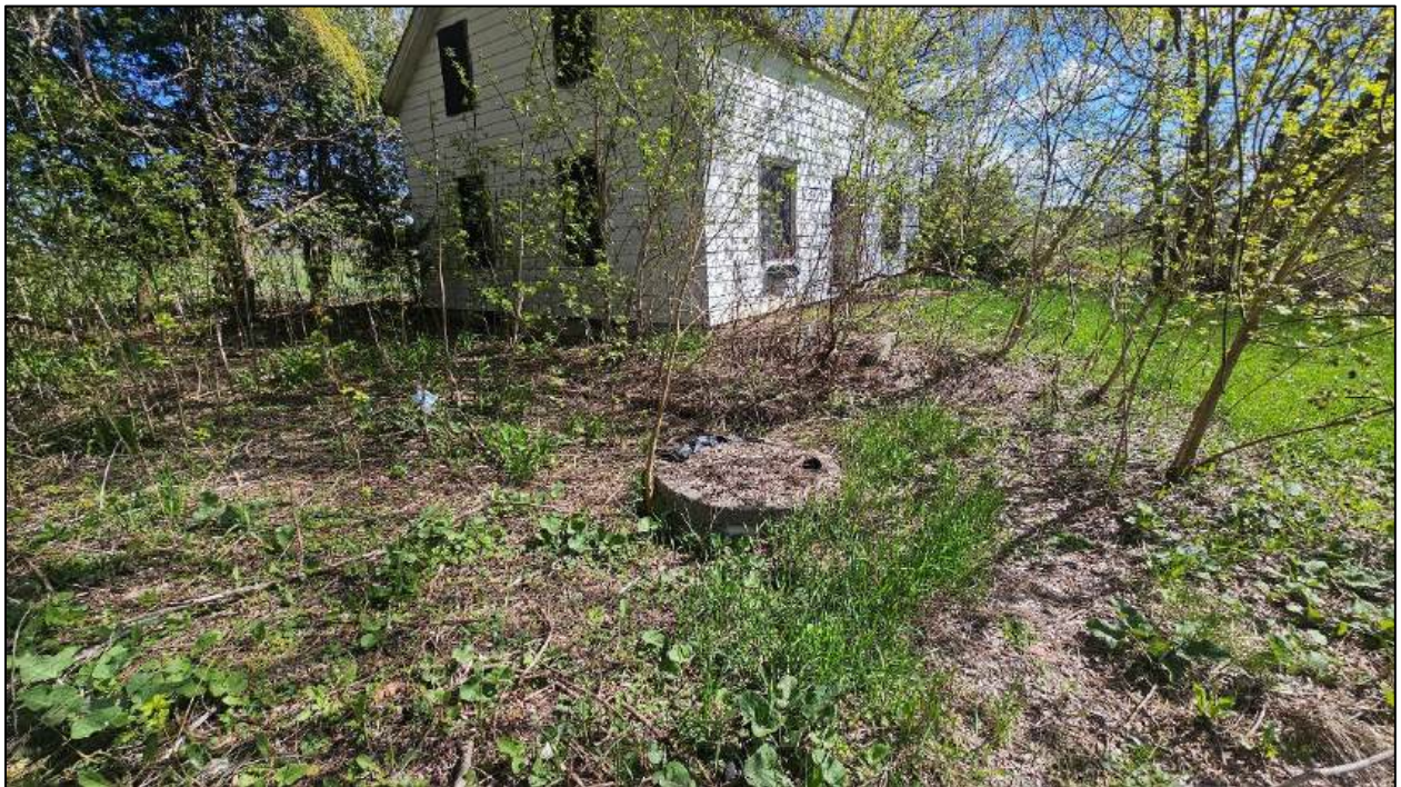
Photograph 12: View of septic pit at 5318 Main Street.
