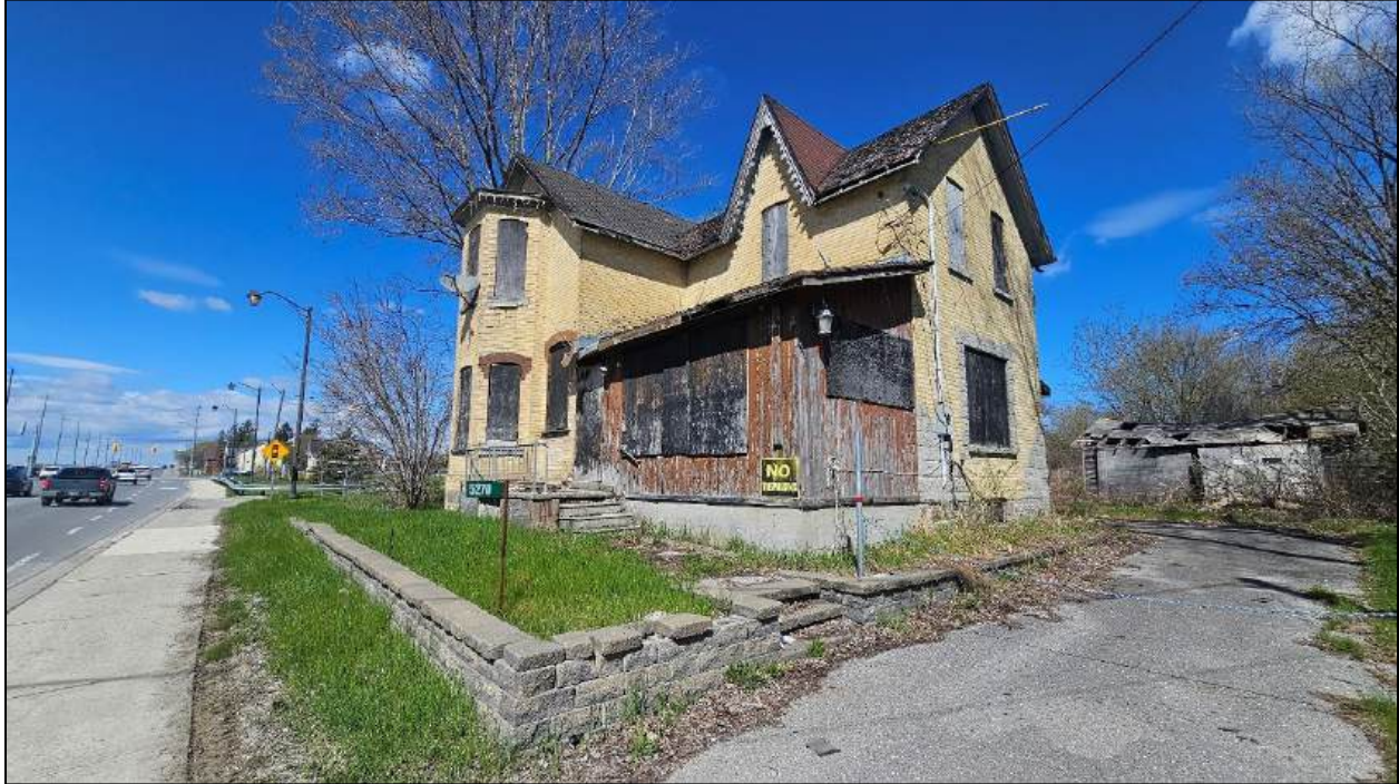
Photograph 3: View of the residential Site building at 5270 Main Street (facing northwest).
