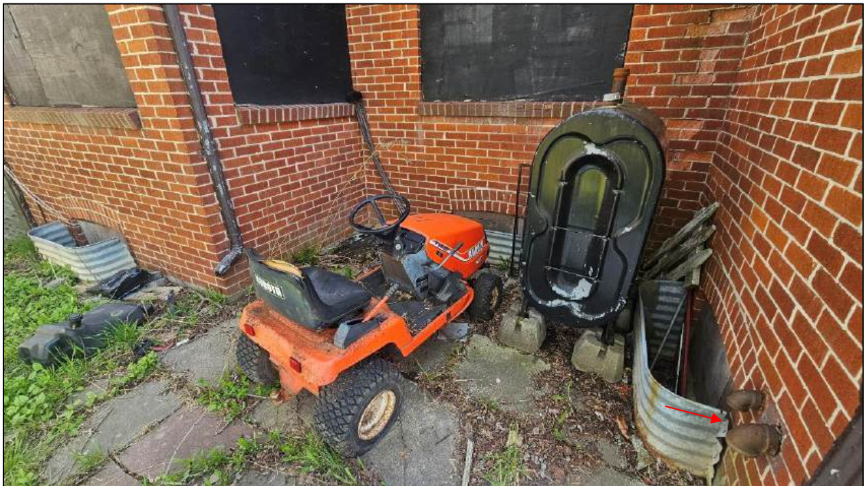
Photograph 16: View of decommissioned AST and cutoff fill/vent pipes observed at 5286 Main Street.
