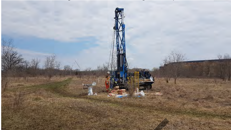
Photo 9 – View of drilling in the central area looking north – April 2019.
