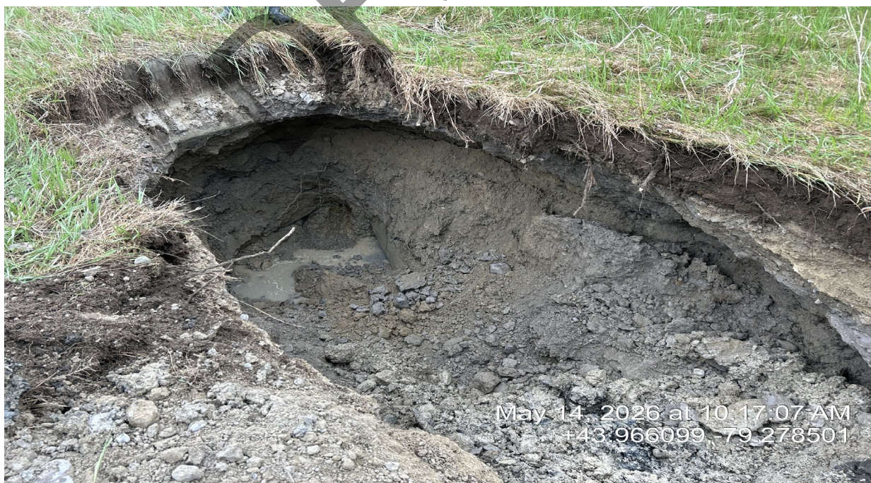
Photo 2 View of shallow groundwater seepage at western portion of the Site
