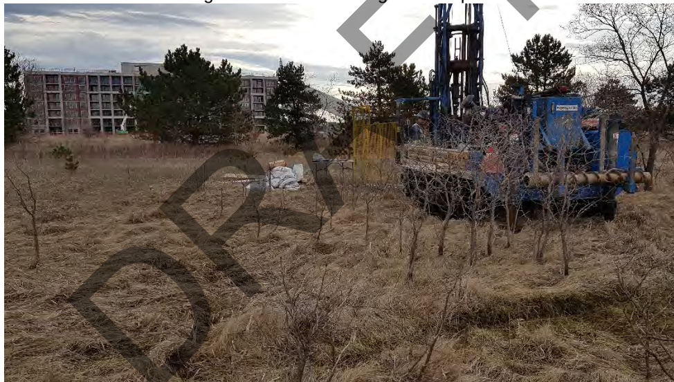
Photo 10 – View of drilling in the central looking east – April 2019.
