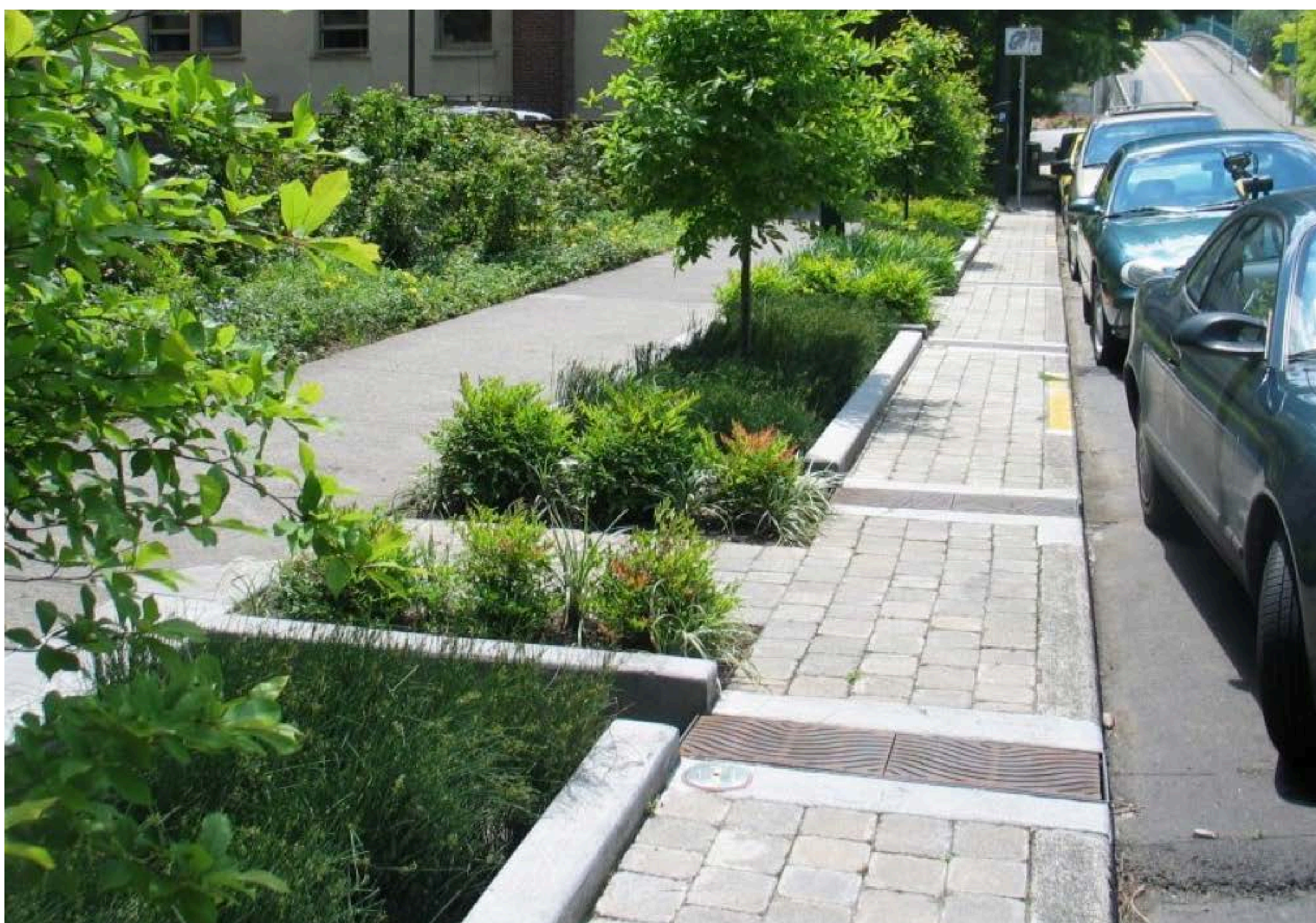
Bioretention tree pit option
