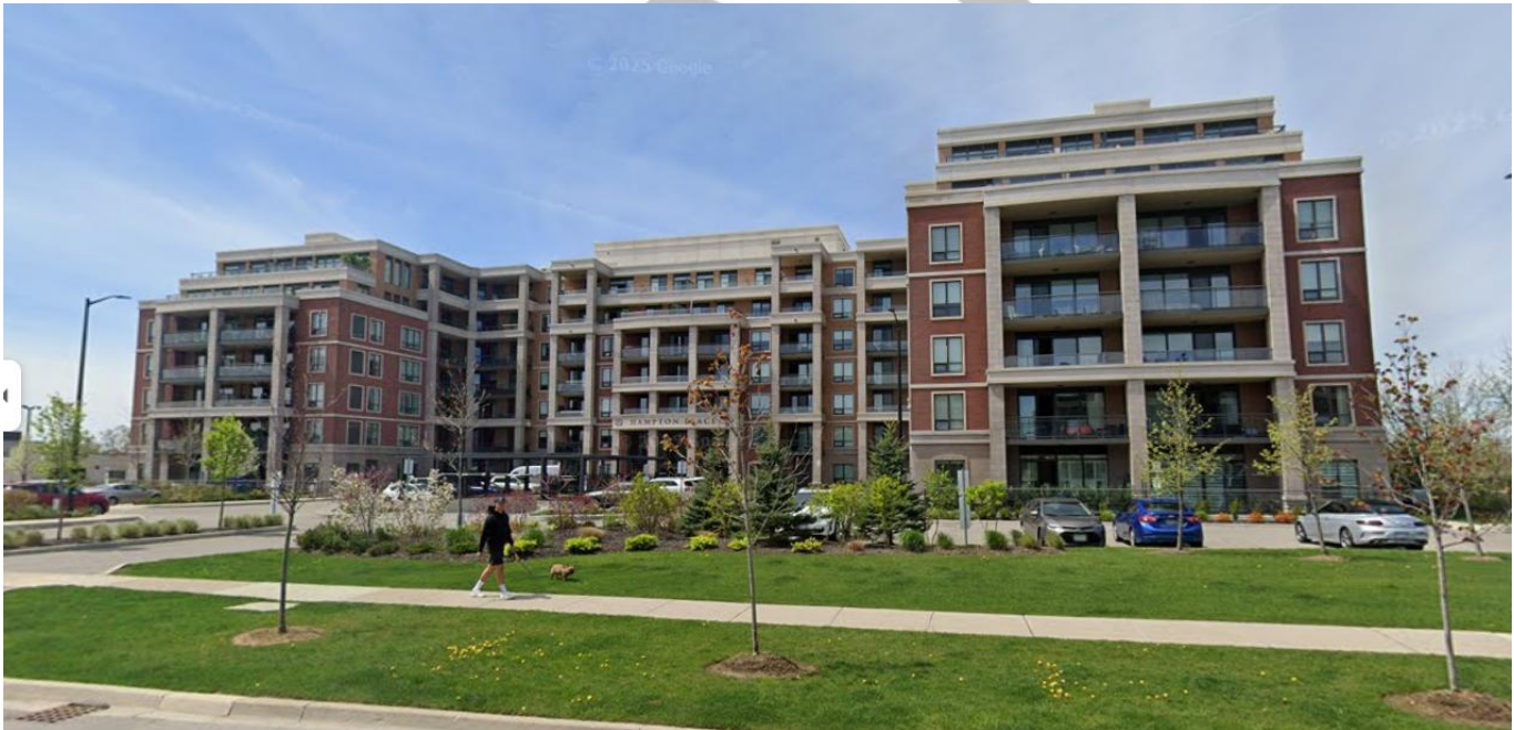
Figure 4 - Zone RN5(3) Example (11750-11782 Ninth Line New Residential) (Source: Google)
