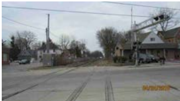
Plate 1: South view of Study Area; Area beyond previously assessed rail corridor is disturbed, no potential
