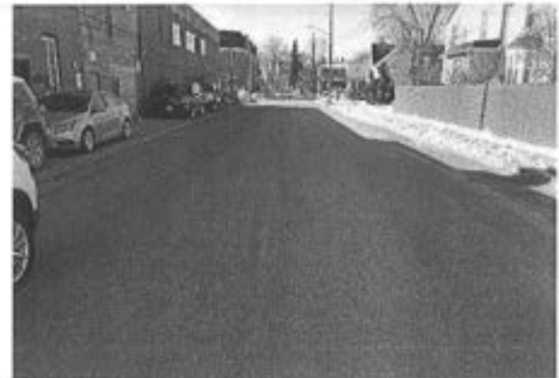
Photo 4: Edward Street looking south, showing the section from Main Street to ~120 m north of Main Street in excellent condition
