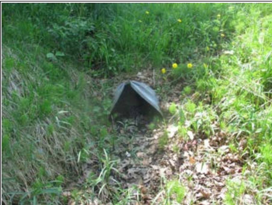
CSP beneath Edward St., E outlet – May 30, 2018
